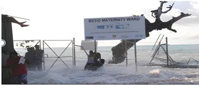
Figure 3 Betio Hospital, Kiribati, during a king tide. (Source: https://www.abc.net.au/news/2016-05-06/fundraiser-launched-to-save-flooded-maternity-ward-in-kiribati/7389670 ).
