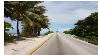
Figure 2 Bridge in Majuro, Republic of the Marshall Islands. The highest point (blue arrow) is less than 10 m above sea level. (Photo: Mai Ling Perman).
