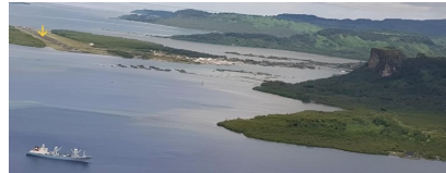
Figure 5 Pohnpei airport, Federated States of Micronesia. The runway (yellow arrow) is within metres from the coast.
